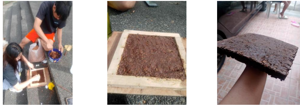
Figure 2. Construction of coconut husk sound absorbing panel.
